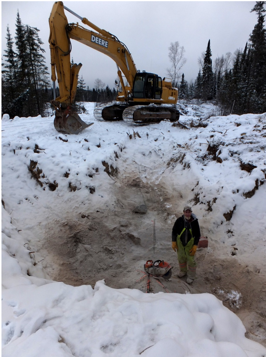
Figure 24: winter trenching program
