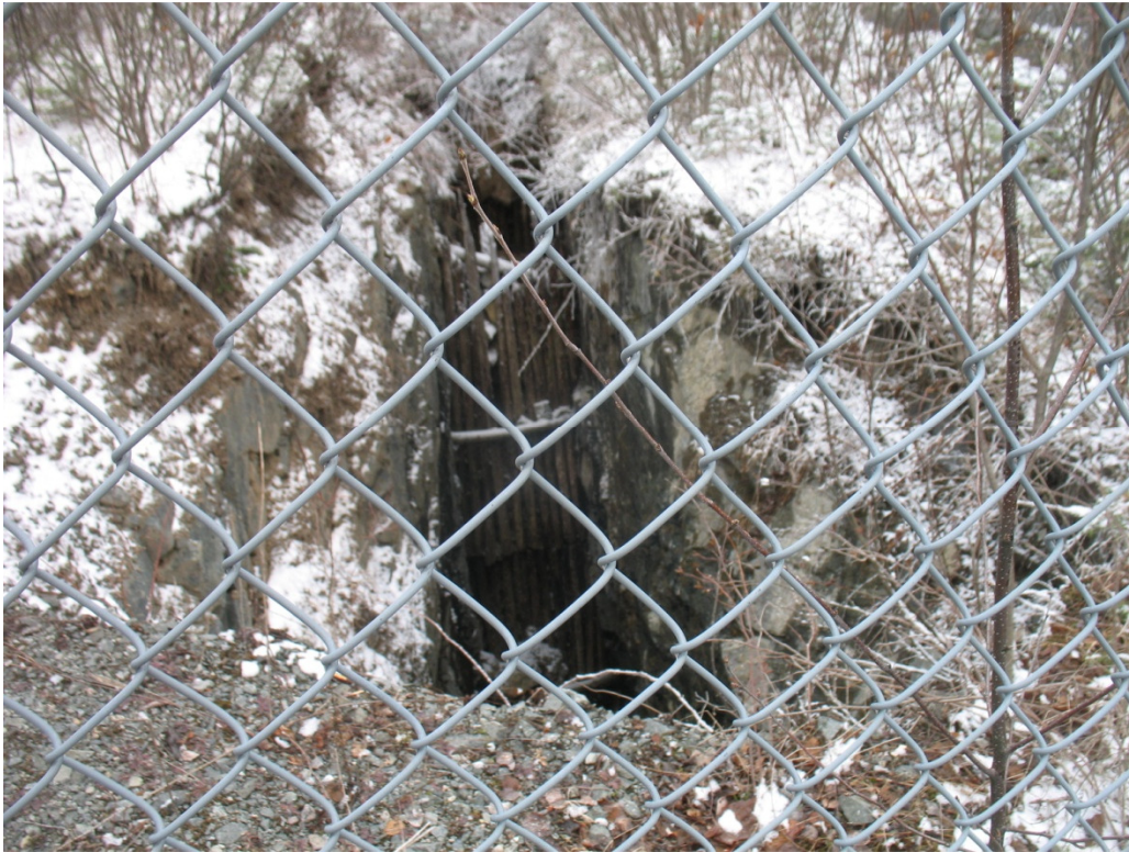
Figure 39 : Rehabilitation and increased safety of the site observed by the QP
