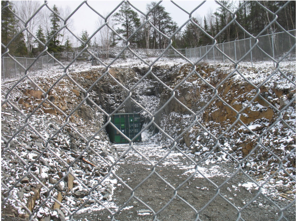
Figure 38 : Rehabilitation and protection of the adit entrance
