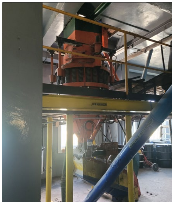
Photo 7: TTL recovery circuit component
