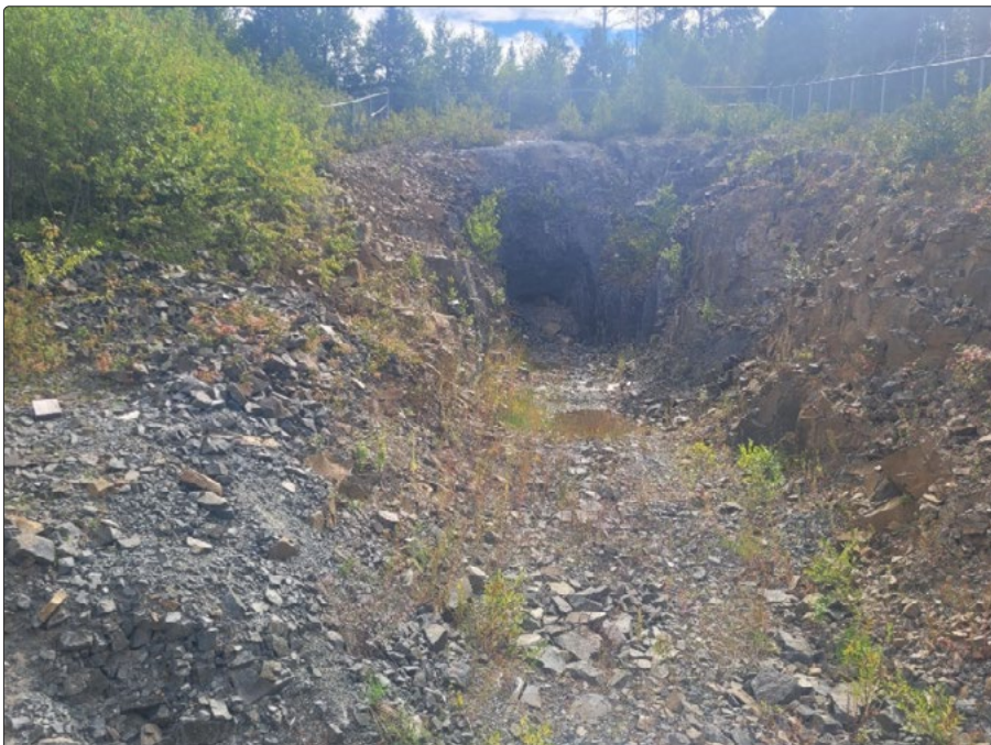
Photo 11: Castle Mine portal
